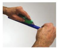
1. Cut and fold back plastic cover to reveal the copper tube
