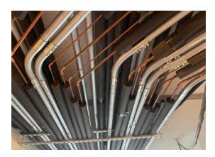
utilized Streamline® Copper Tube as well as over 1600 size 1/4" - 3/4" Streamline® ACR Copper Press Fittings and CYCLEMASTER® FTG x FTG Multi Split Ball Valves to complete the building's VRF system installation.
