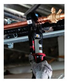
We are proud to have partnered with Milwaukee® Tool in the development of proprietary jaws for use with our dual-seal Streamline® ACR Copper Press Fittings. These proprietary jaws are compatible with most common standard full-sized press tools on the market.
